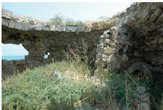
Figure 13 – Location A, Prior to excavation, General view.
