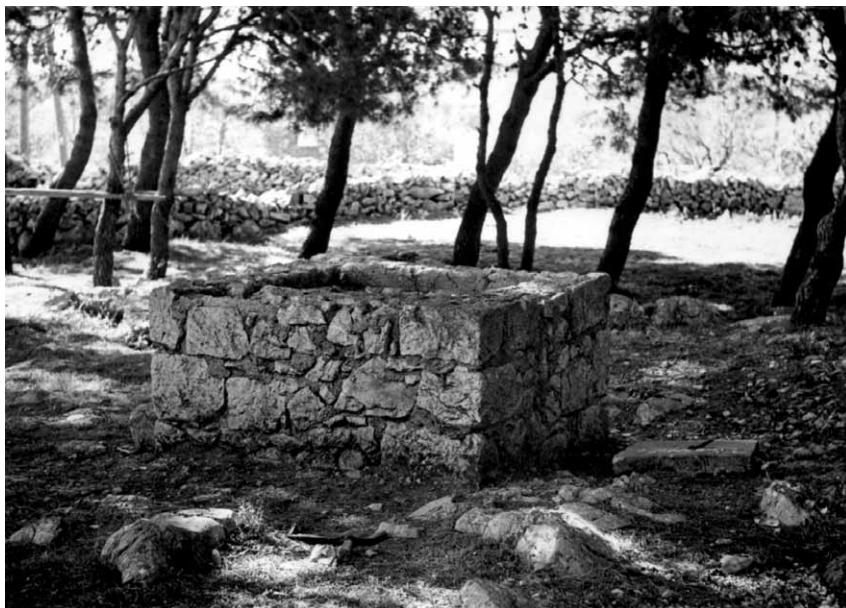
Fig 15 – Wall around the shaft O-7 (B. Ilakovac).
