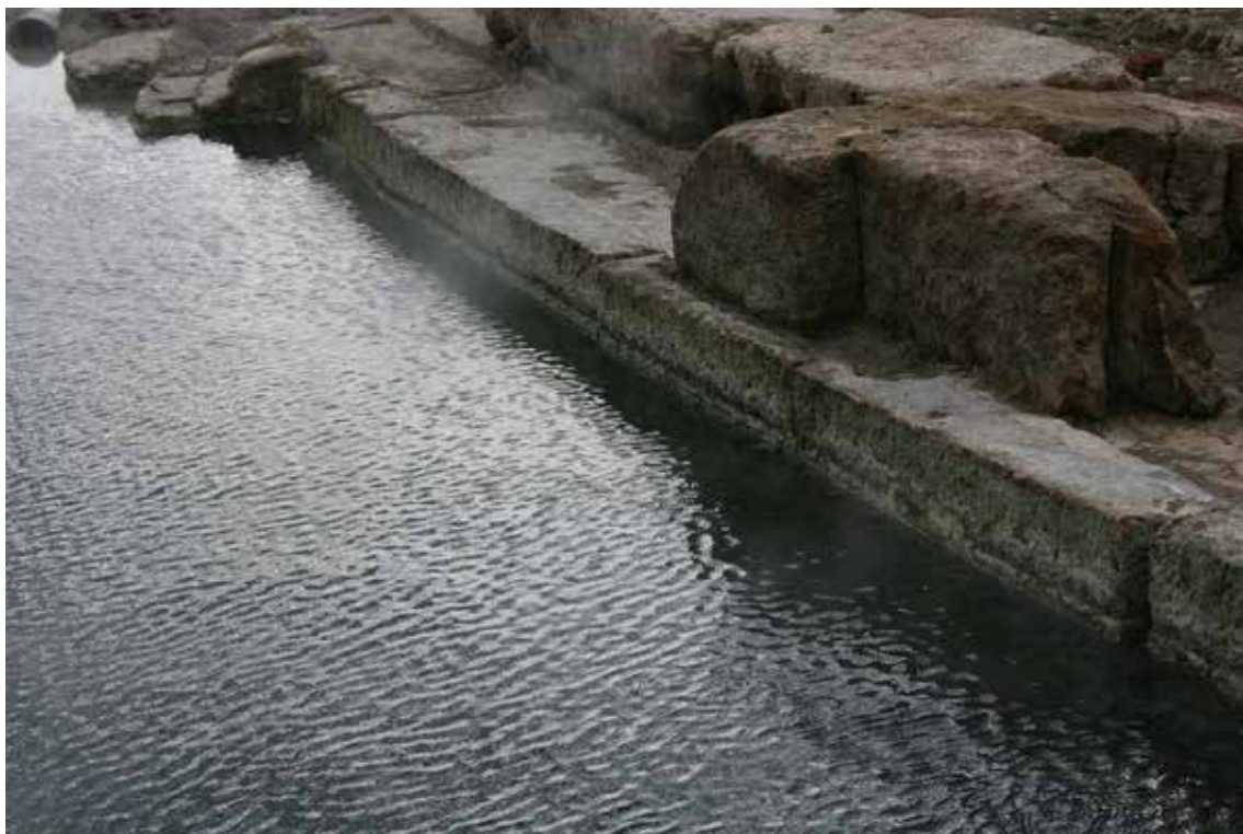
IZVORIŠNI BAZEN - ZAPADNI ZID (2. – 4. st.) SPRING POOL - WEST WALL (2 nd –4 th centuries)
