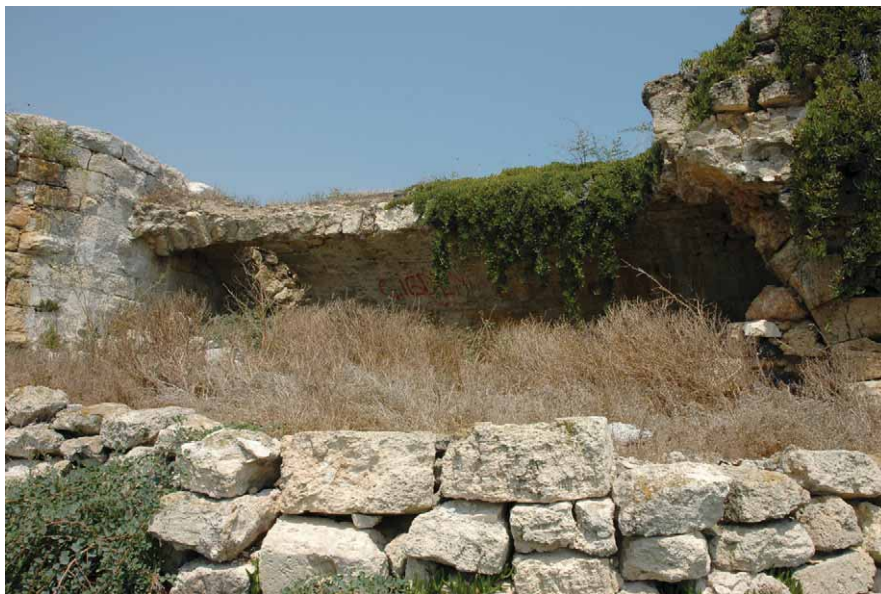
Figure 15 – Location B, West side, prior to excavation.
