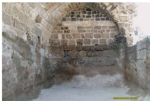
Figure 25 – Location B, After excavation, View to the west.
