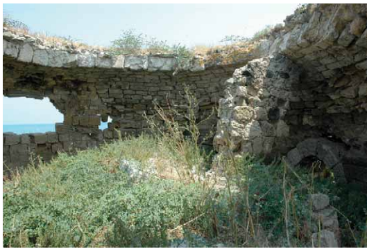
Figure 13 – Location A, Prior to excavation, General view.
